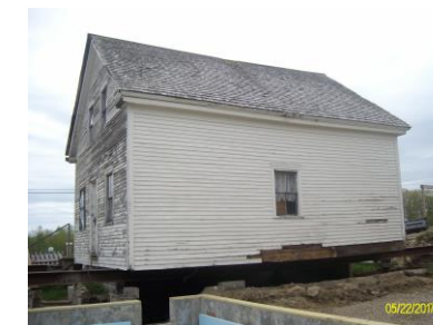
Peter Field House Renovation
