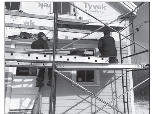
Work continues on the clapboard siding of the Fields House.
