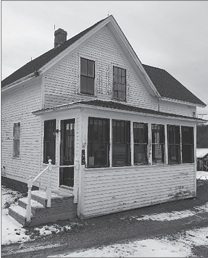
Curran farmhouse. A new roof was recently installed on the farmhouse thanks to a generous donation from Irv & Karen Marsters. Further repairs will proceed in the spring including a new coat of paint for the structure destined for greater activity in 2020 starting with our Cabin Fever Workshop series (see details).
