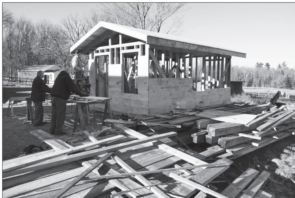
Post Office building under construction.
