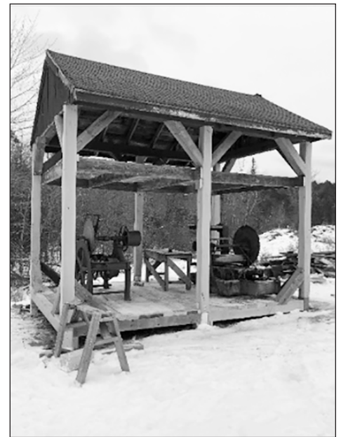
Single Mill Shed
