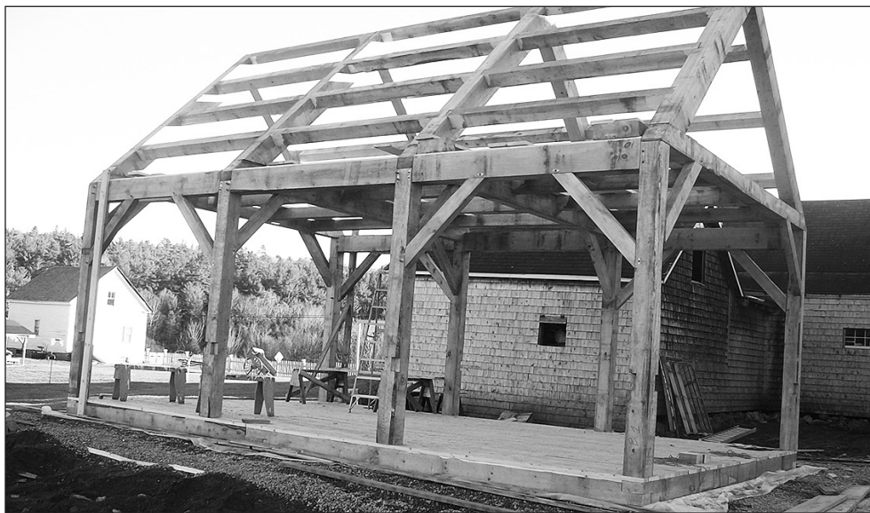
Our first mortise and tenon workshop produced the framework in part for our Carpenter Shop.
